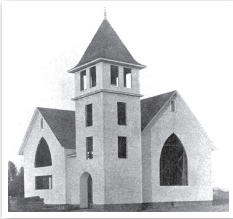
Construction of the First Mennonite Church, 1908. (Photo courtesy of First Mennonite Church Archives.)
